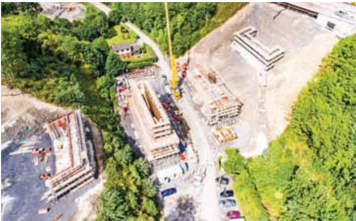
Bridge S5 – Middle Dolfor Lane
