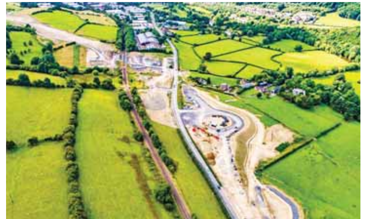
Pool Road tie in works
