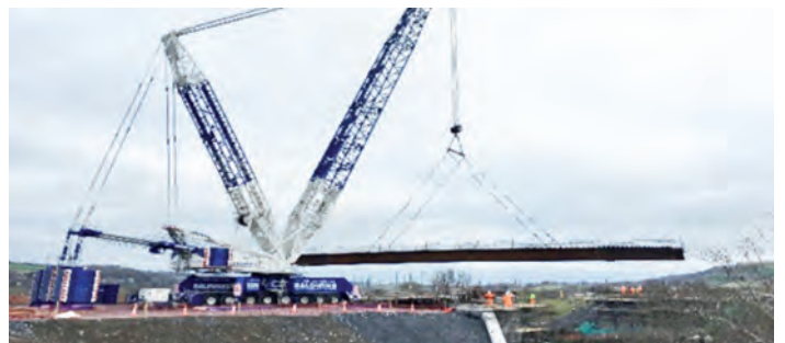
Pictures of crane lifting operations at Mochdre Bridge
